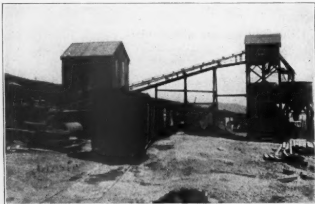
The 57th Street Plant
